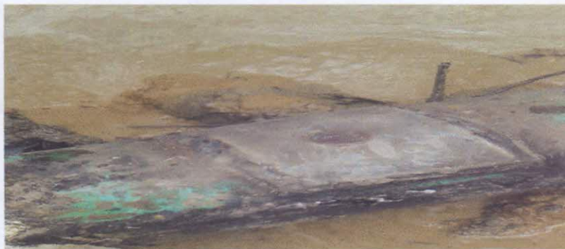
Point after repair.
