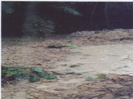
Point after barricading to expose pipe.
